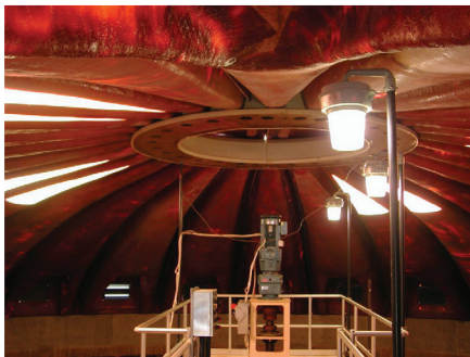
Interior View of Dome Cover System
